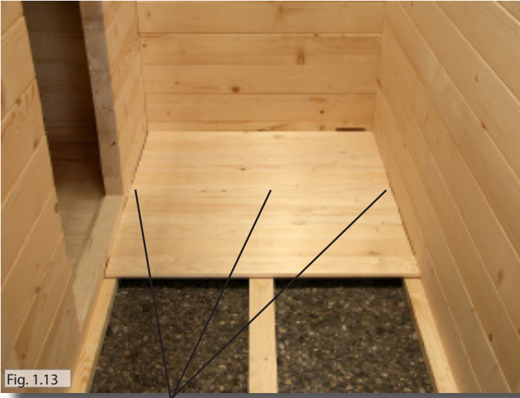
Floor - screws 3.5 x 50 mm
